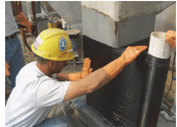
Fig. 2. Fragment of work on the reinforcement of columns with
