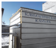
Fig.1 - General view of the climate chamber.
