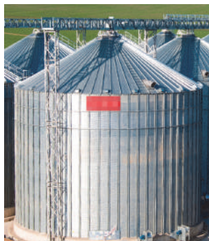
Fig. 1 – General view of grain drying complexes
