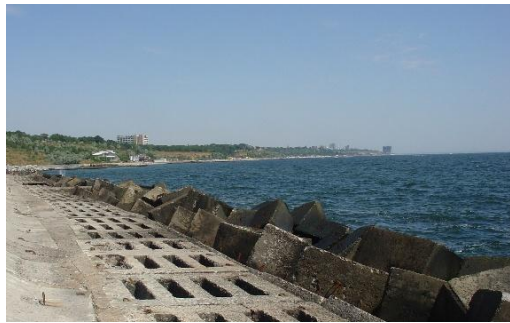
Fig. 4. Shore protection in the area of Cape Velykyi Fontan, Odesa
